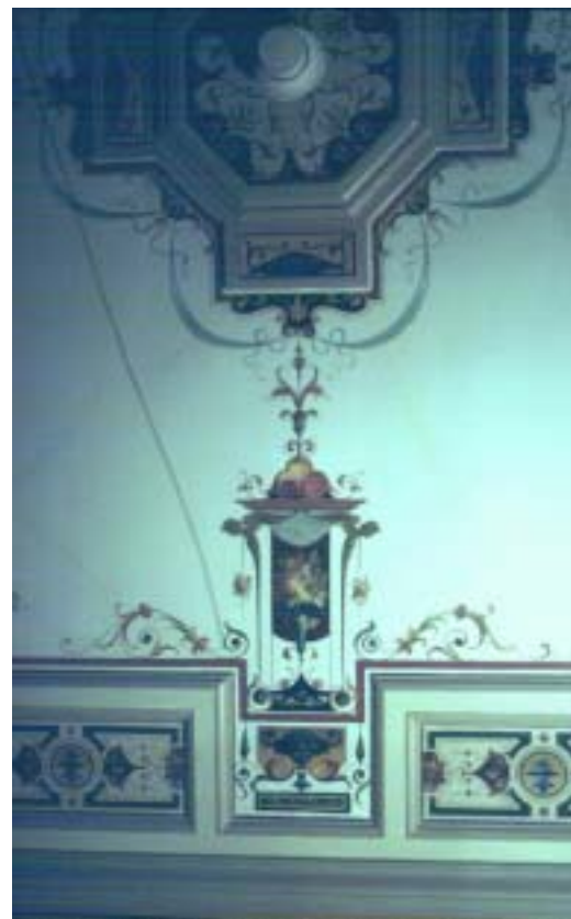
Abb.366 VILLA Rieter, Bad Decke Detail
