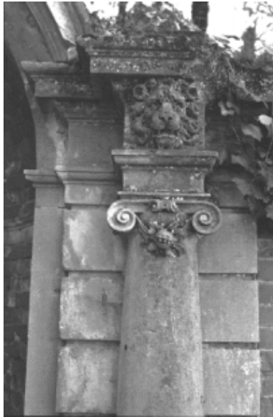
Abb.363 VILLA Rieter, Brunnen Detail
