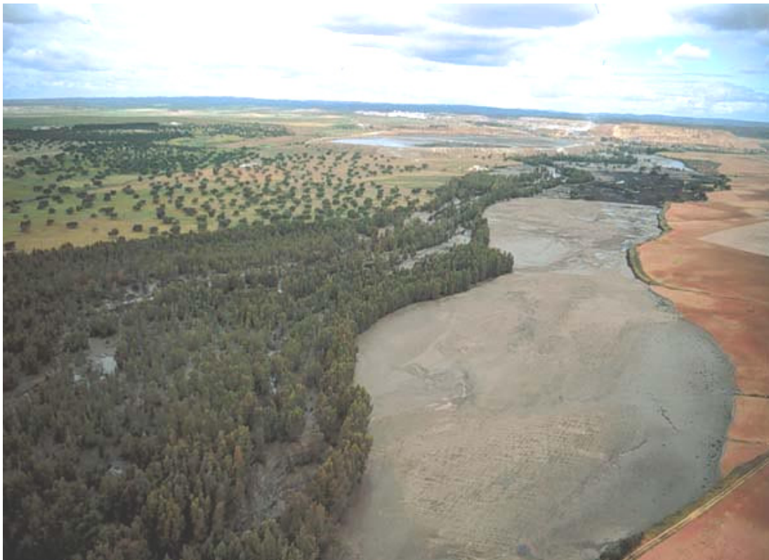
Figure 3.6. Aerial view of Rio Agrio floodplain after the accident. View to NW (from Aguilar et al. 2000)
