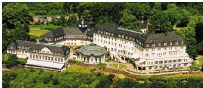
Figure 2-5: picture of Steigenberger hotel in Switzerland
