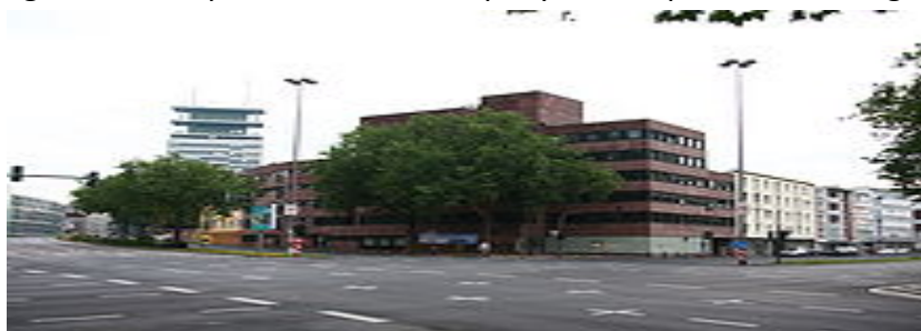
Figure 2-12: A picture of HRS company's headquarters in Cologne
