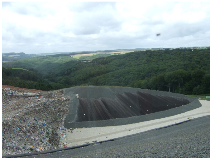
Figure 4.6: Landfill covered with asphalts at Fridhaff-Diekirch
