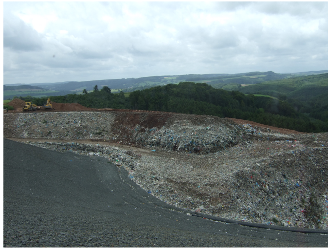
Figure 4.5: Condition of disposal site at Fridhaff-Diekirch
