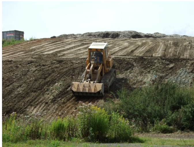
Figure 4.10: Condition of disposal site at Linkenbach
