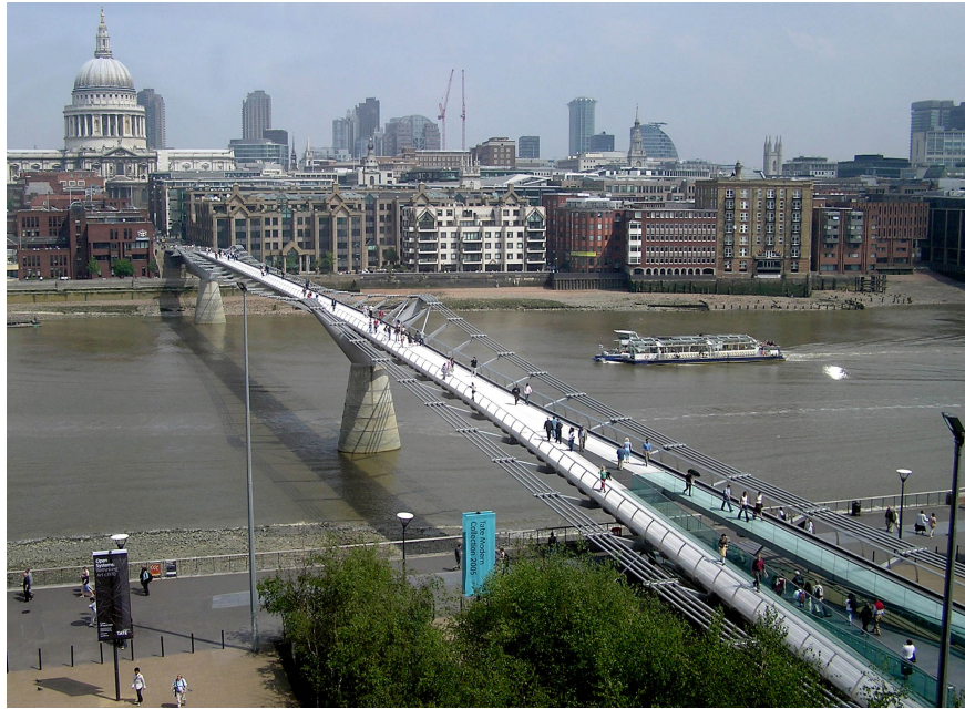
Figure 1.2: Millennium Bridge in London, Image Courtesy of Wikimedia Commons
