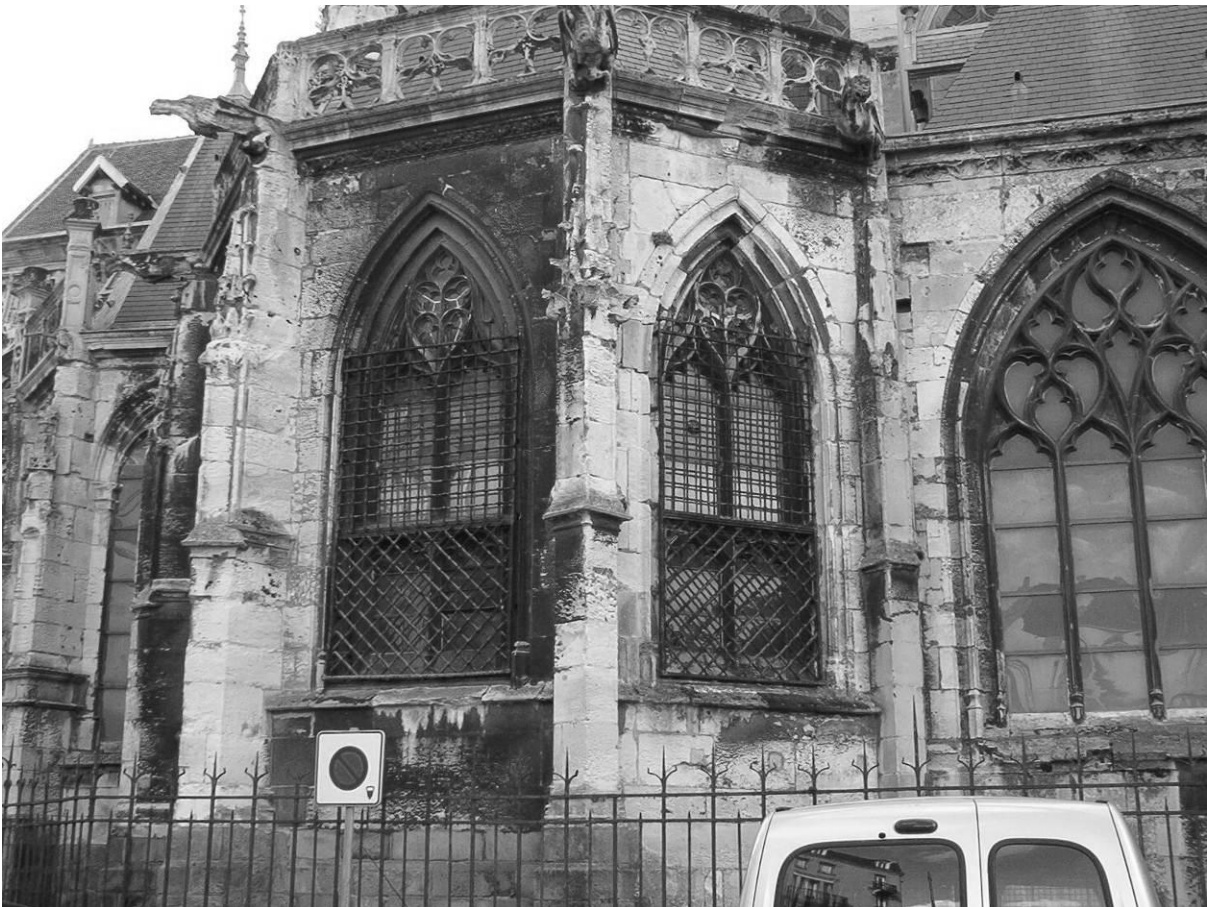
Abb. 246: Dieppe, Saint-Jacques, Sakristei v. NW., Fenster
