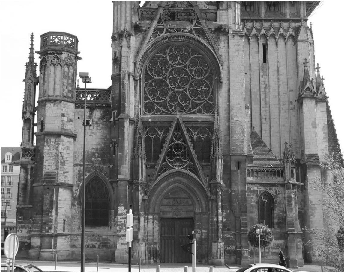
Abb. 7: Caen, Saint-Pierre, Westfassade v. W.
