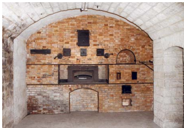
Foto 26: Backofen (Fort Sucty, Ile-de-France)
